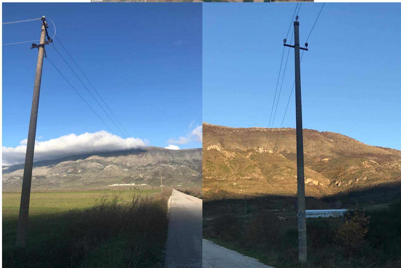
Figure 29. Gline-Drino valley power line recommended for insulation and installment of bird diverters
